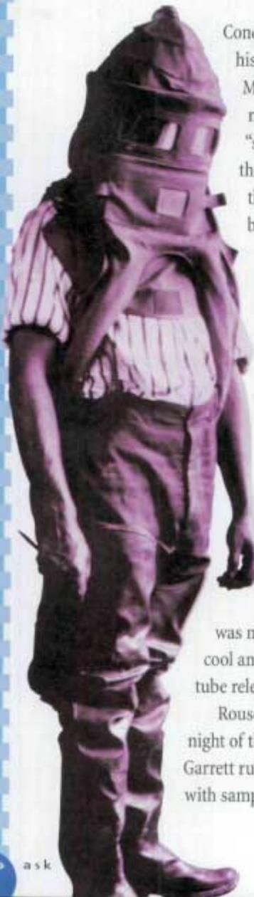
Concerned about his employees, Morgan experimented with a "safety hood" that would allow the wearer to breathe despite a fire's toxic smoke. Morgan knew smoke rises during a fire, so he created a heat-resistant hood with a long tube reaching to the floor. Wearing Morgan's hood, a firefighter could breathe the cleaner air near the ground. Morgan lined the breathing tube with a sponge-like material that was moistened before use to cool and filter the air. A second tube released exhaled air.
